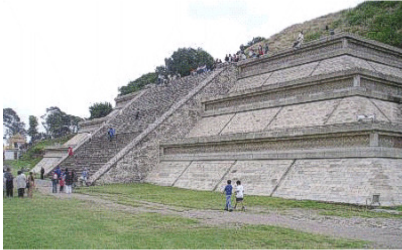
Small portion of a staircase on the side of the Great Pyramid of Cholula, Mexico
